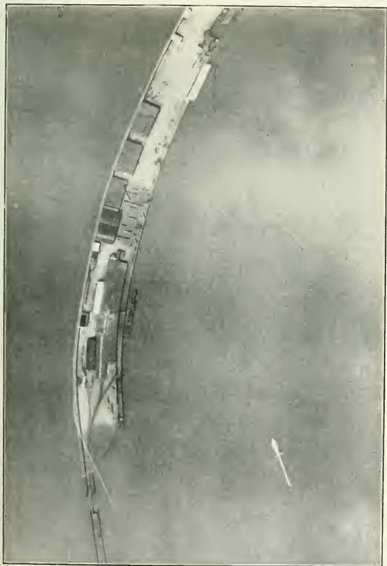
SEA-PLANE VIEW OF THE MOLE, SHOWING THE VIADUCT REPAIRED
